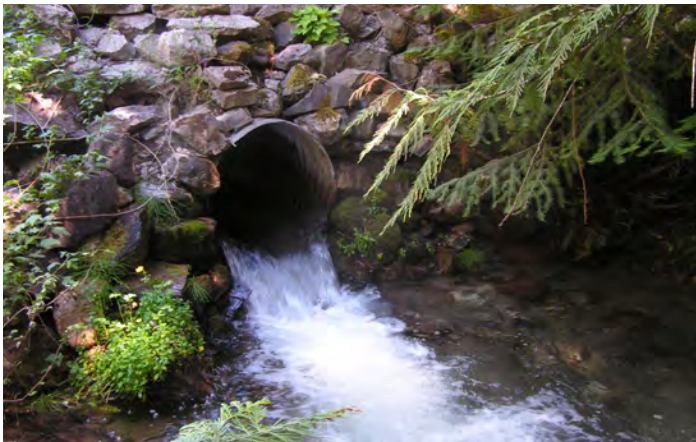
Example of a culvert that blocks fish passage and doesn't facilitate movement for terrestrial wildlife. Photo courtesy of Washington Department of Fish and Wildlife
