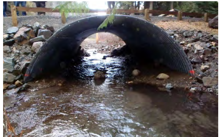
An aquatic organism passage (AOP) culvert that facilitates movement for fish and other species such as frogs, salamanders, small mammals, insects, and microorganisms
