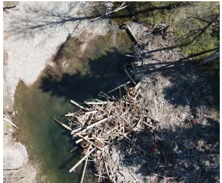
An engineered logjam on the Cispus River
