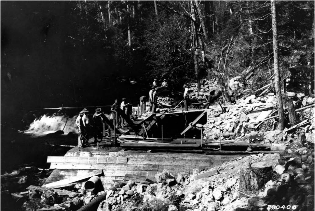
Members of the Civilian Conservation Corps building a dam on Trout Creek in 1933
