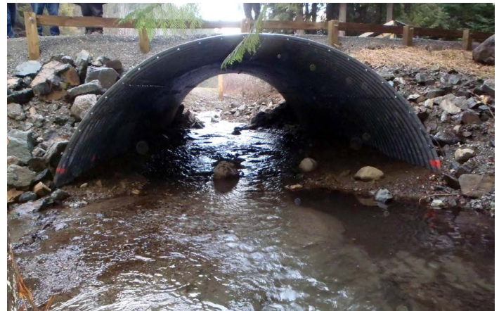
An aquatic organism passage (AOP) culvert that facilitates movement for fish and other species such as frogs, salamanders, small mammals, insects, and microorganisms
