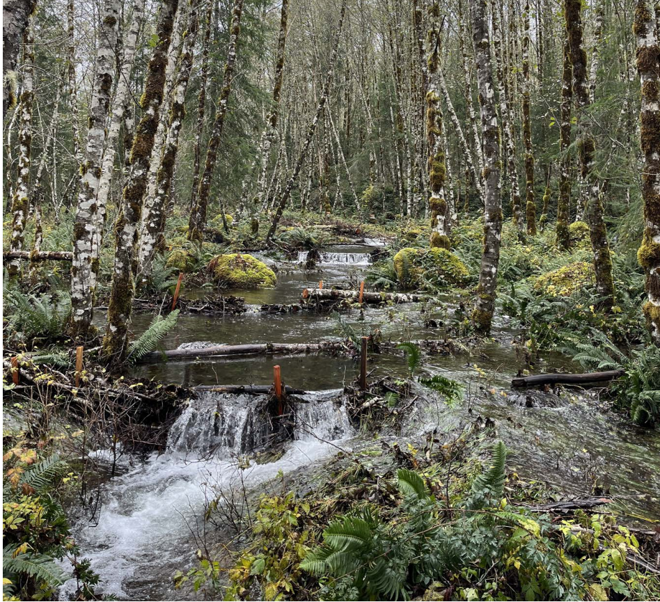
Beaver dam analogs installed by CFC and volunteers along Stump Creek
