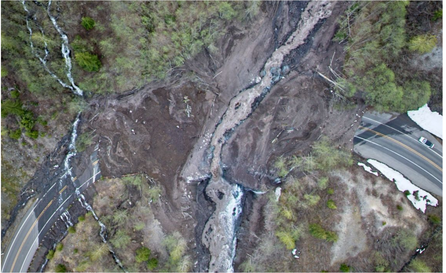
Washout on route 504 near Mount St. Helens. Photo courtesy of Nickolett Uhler and KGW
