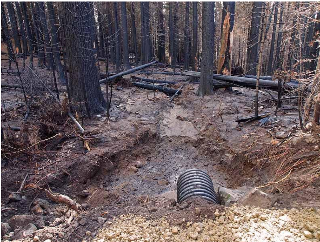
Photo #1: Culvert in Unit 6, post rocking and clean up.
